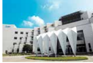
Tainan Plant (Diamond-rated Green Building)
